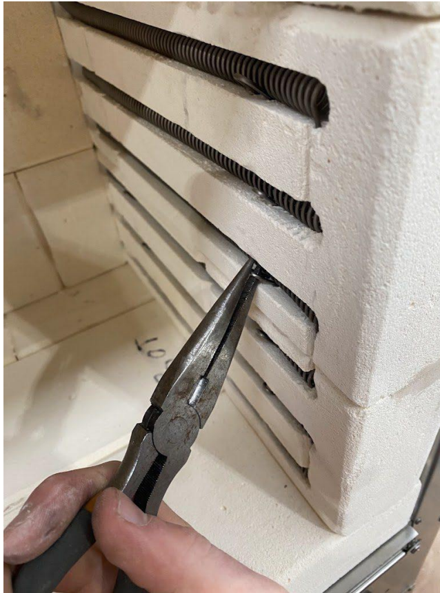
Pushing a FeCrAl staple pin straight into the soft brick with long-nose pliers, so the bridge holds the element down in its groove. No drilling is required.
